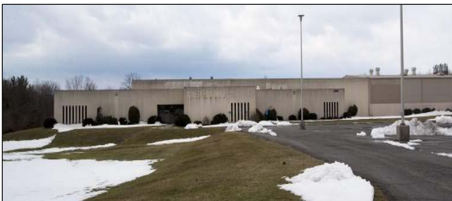
3085 Shawnee Drive—the Site of our Future Home
